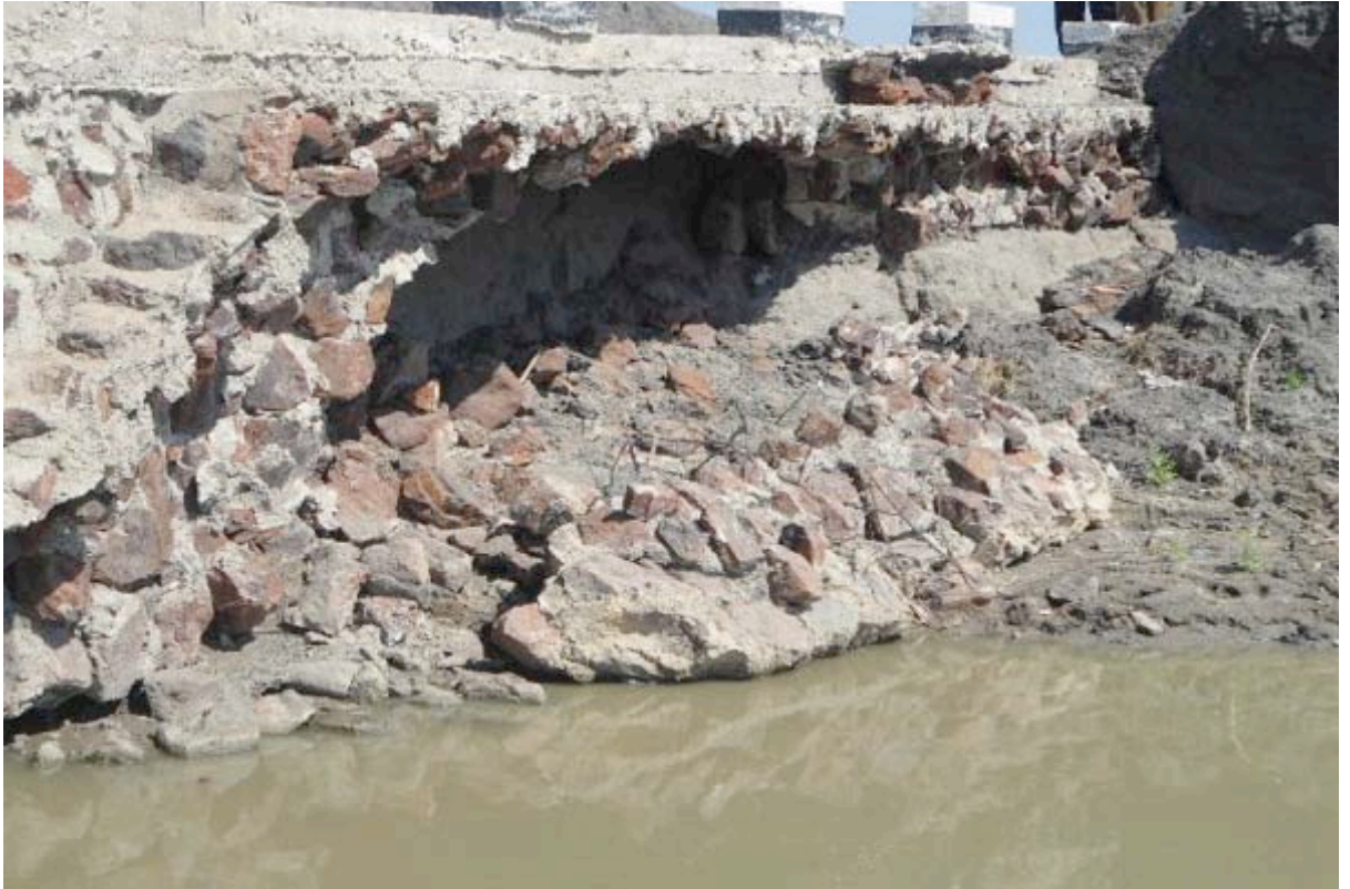
Poorly designed drift
