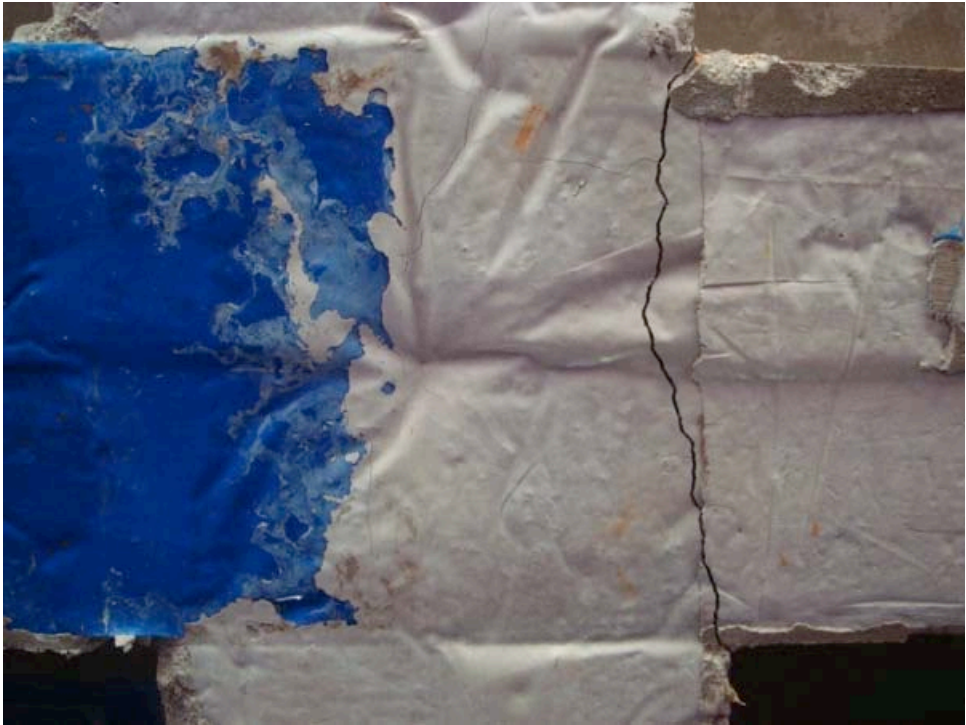
Beam failure on a recently constructed bridge
