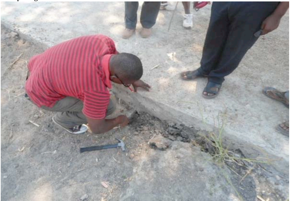
Auditors checking the recently constructed drift
