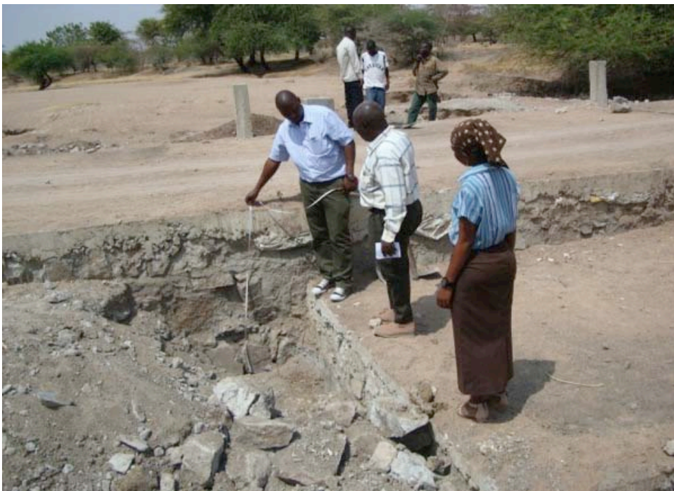
Shallow constructed cut-off wall
